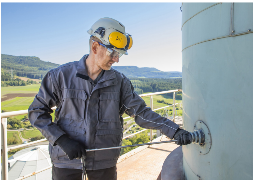
Figure 4. Regular monitoring using the testo 350 exhaust gas analyser allows for the optimisation of combustion parameters and processes conditions.
