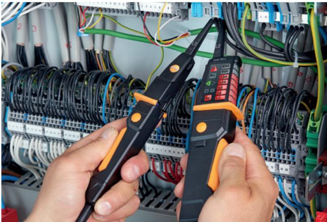
Measuring voltage in a switching cabinet.
