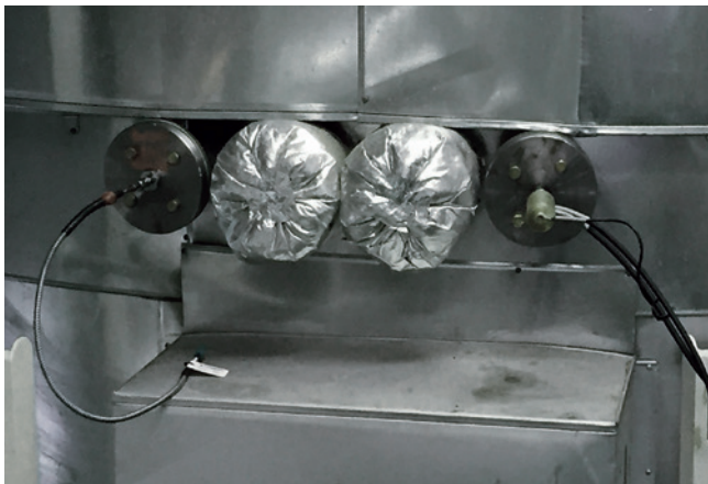
testo 350 probe fixed to the measurement site with a flange.
