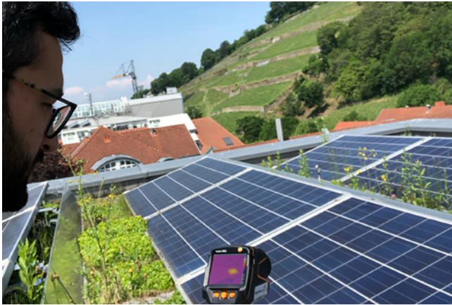
Figure 3: The testo 883 thermal imager in use inspecting a PV system.
