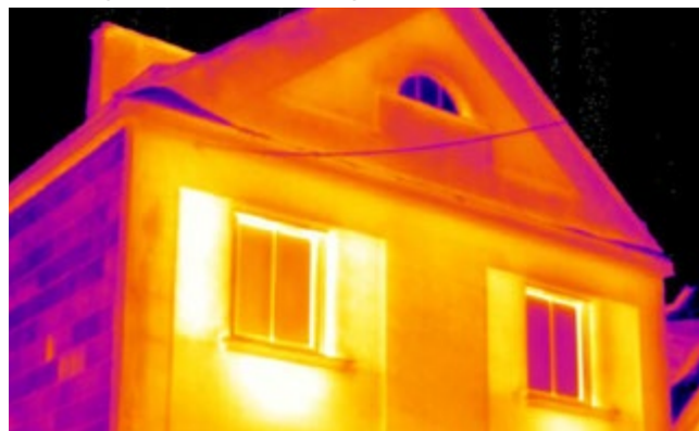
Carrying out detailed energy consultancy
