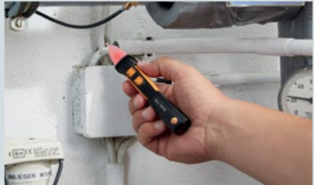
Non-contact voltage testing on a distributor box with the testo 745.
