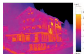
Thermal image with ScaleAssist
